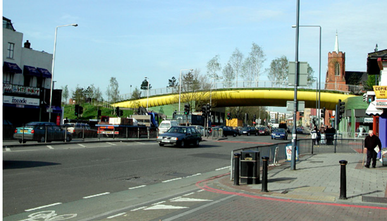
The Green Bridge
